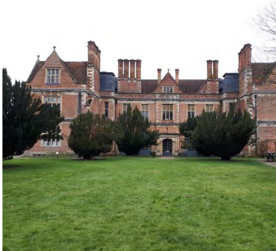
Figure 6.1 Grade I listed Shaw House
