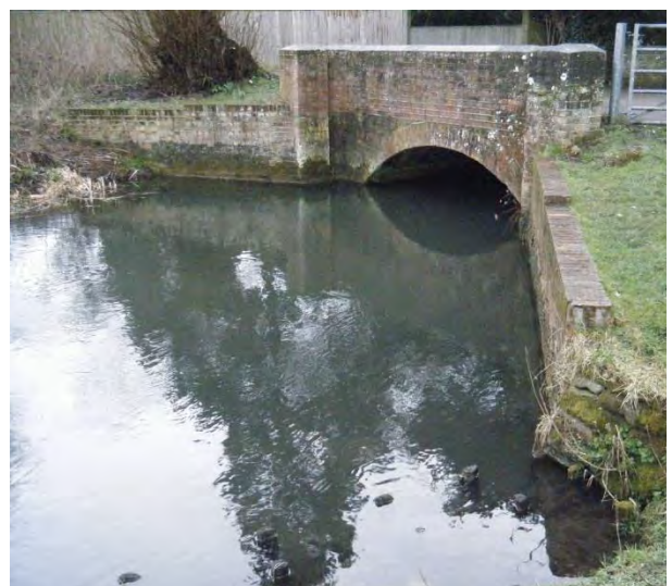
Figure 6.6 Unlisted bridge over the River Lambourn
