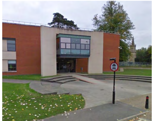
Figure 6.4 Trinity School buildings
